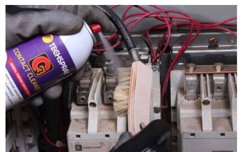
Step 2: Remove grease and sludge with aerosol cleaner
